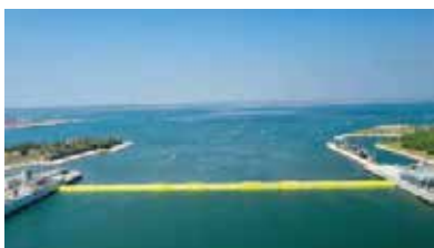
Process and Fire Pumps for MOSE Flood Control
